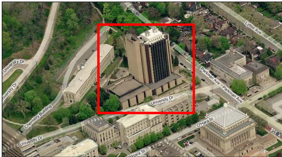
Figure 2 Bird's Eye View of the Chevron Annex and adjacent structures prior to construction
